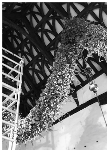
Right: The Garland under construction with only the far side completed.
